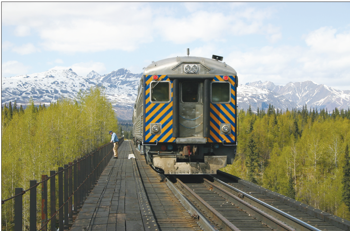
Hurricane Gulch Bridge: Northern turning point for the Hurricane Turn service
